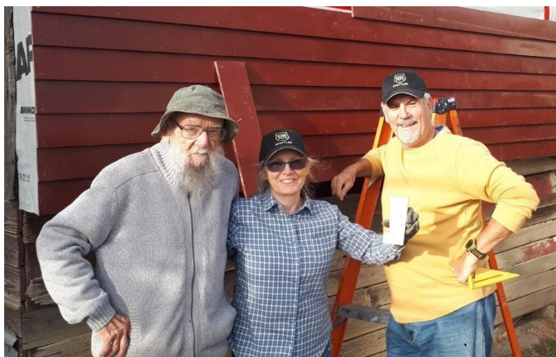
Frank Hackler, Carol and James Hall installing siding on Feed Shed
