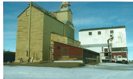
Feed Mill Wall Repaired Summer 2010
